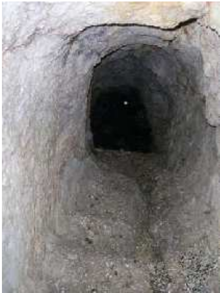
Galería de la mina (D. Ortiz, 2012)
