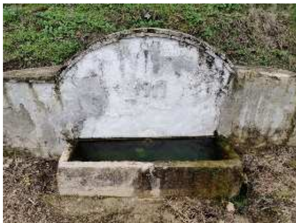
Pilar de Sales (D. Sánchez Garrido, enero 2022)
