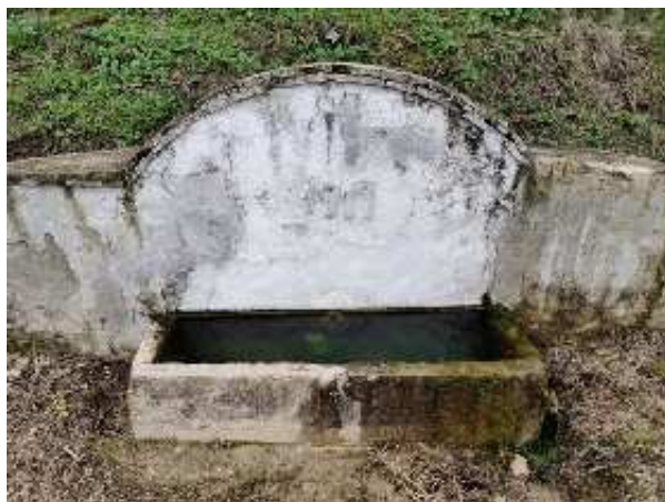
Pilar de Sales (D. Sánchez Garrido, enero 2022)
